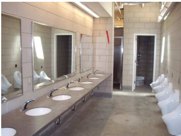
Men's Restroom approaching completion
