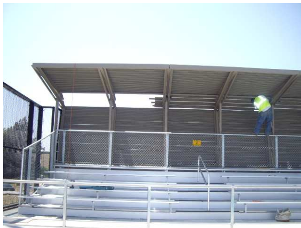
Roof for bleachers is being finalized.
