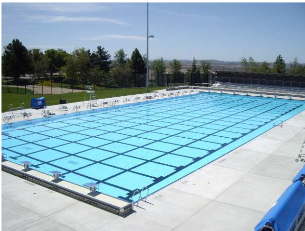
Myrtha Pool completed & filled with water
